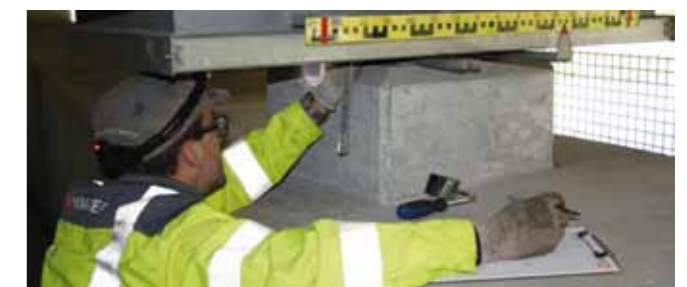
Inspection of bridge bearings
