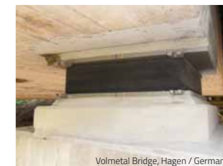
Volmetal Bridge, Hagen / Germany
