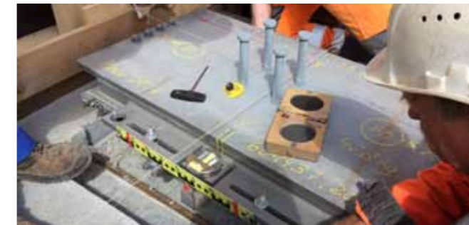
Installation Botlekbrug, Netherlands
