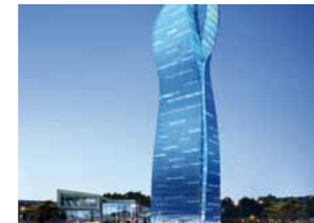
TUNED MASS DAMPERS
